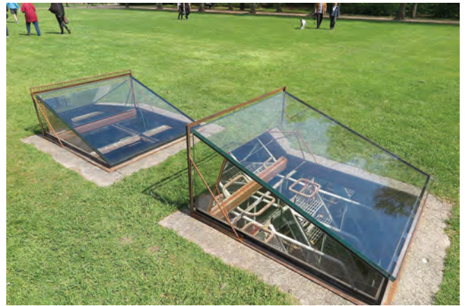
The emergency exit from the Cistern in Søndermarken Park in Copenhagen. The glass roof provides light to the art installation below, where moss and other plants currently grow within the reservoir
